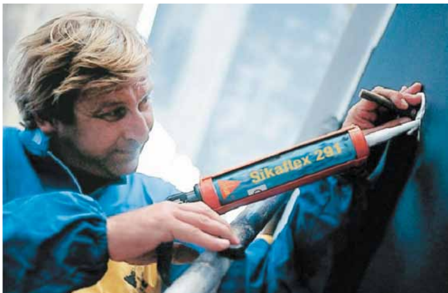
Fig. 80 Sikaflex®-291 is applied
