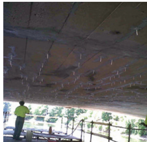
Epoxy injection of arch ring
