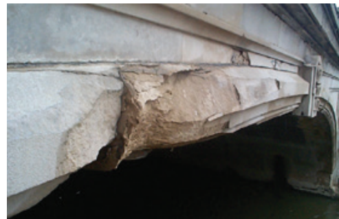
Spalling of the stone façade on the arch ring
