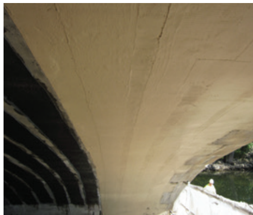
Partially completed installation
