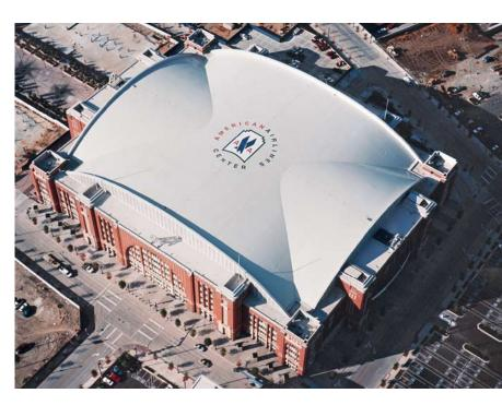
Developers of the American Airlines Center in Dallas, Tex. appreciated the design flexibility and durability of a vinyl membrane for the facility's 200,000 sq. ft. of multi-sloped roofs joined at right angles. The tan coloring matched the exterior façade's Indiana Limestone and GFRC; separately, vinyl film membrane for the custom logo was welded directly onto the main membrane.
