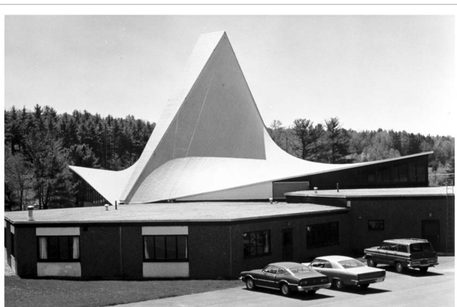
First United Methodist Church in Gilford, New Hampshire, Installed in 1976
