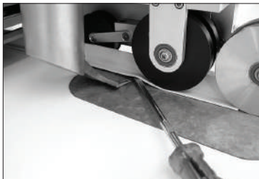
Fig. 1.8 Lifting the rib to insert the Sarnamatic nozzle
