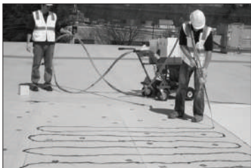
Cart and hose application
