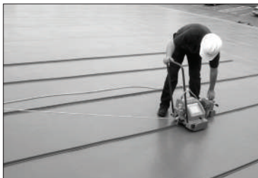
Fig. 1.5 Safety rope securely attached to the Sarnamatic
