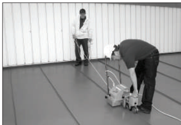
Fig. 1.9 Guiding the Sarnamatic along the correct line
