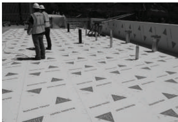
Vapor Retarder SA 31 cut tight around penetrations
