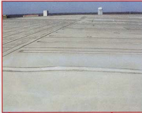
Photo 7: Partially deformed fixation bar.
