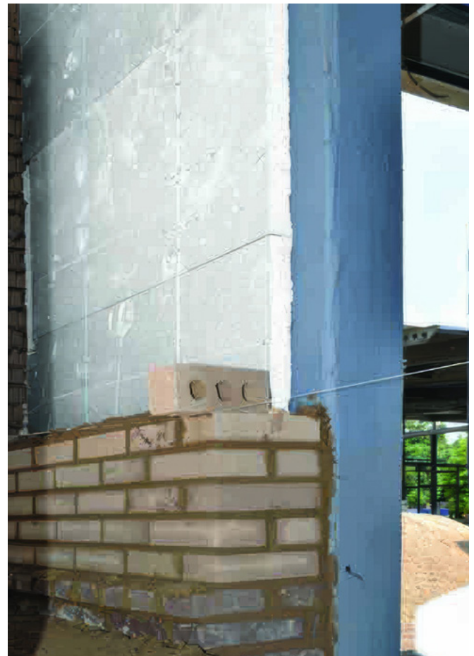
WeatherSeal air/water-resistive barriers can provide a continuous air and water-resistive barrier behind multiple claddings for uninterrupted air and moisture protection
