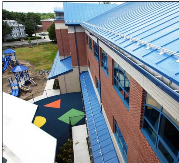
Décor Profiles, or "Ribs," give the vinyl roof the look of standing seam metal. The Profiles have the same product formulation as the membrane, ensuring that colors will match, both initially and over time.
