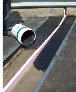
Install into blockout
