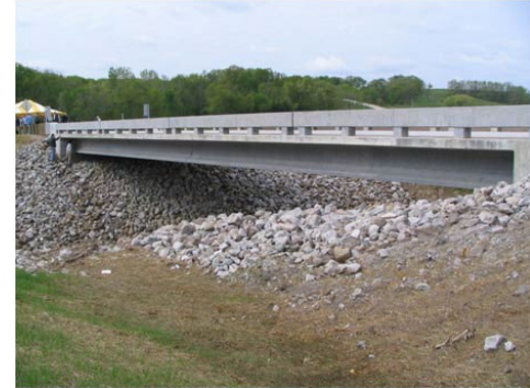
Mars Hill Bridge (Wapello County, Iowa) 110 ft girders with no rebar for stirrups
