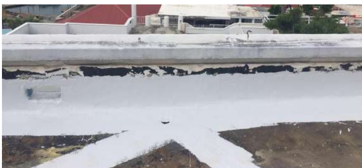
RoofPro detailing at scupper and 90-degree joint at parapet wall.
