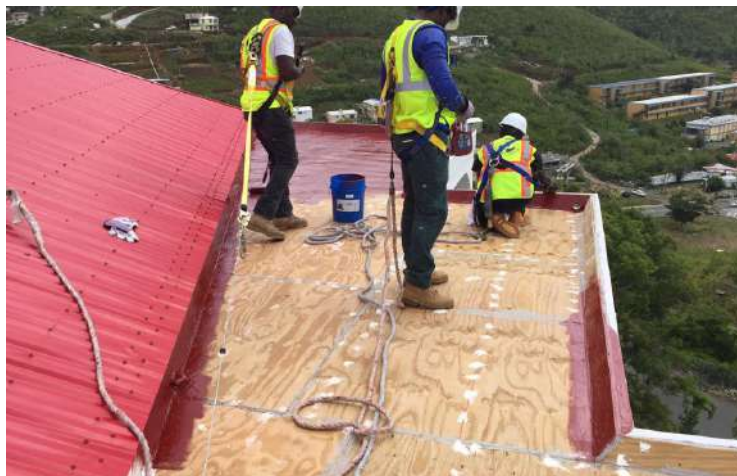
Sika EP epoxy primer application on plywood deck.
