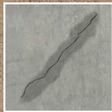
Leaking cracks
