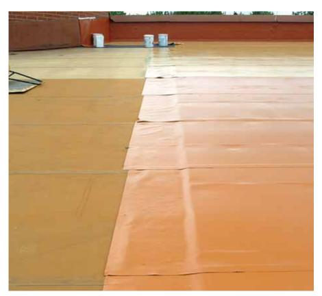
Because of this roof's high visual profile, one small wrinkle or patch in the finished fully adhered surface would have completely ruined the effect of the multi-colored membrane, so the "lawn-rollered" application had to be perfect, creating a real challenge for installers. (Photos courtesy of Sarnafil Inc., Canton, MA.)
