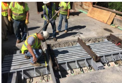
JOINT SEAL ASSEMBLY
