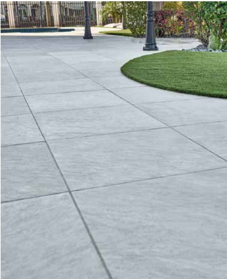
Merkrete Underlay C flattened surface irregularities and established proper slope for drainage.
