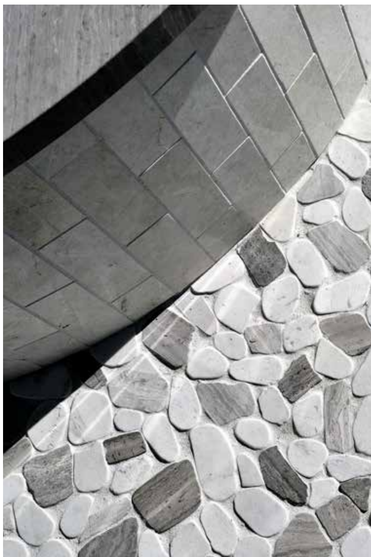
SikaTile®-815 Secure Grout fills the space between the pebbles surrounding the firepit.
