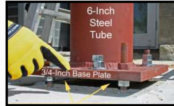
Void is filled with Sikadur 32 Hi-Mod
