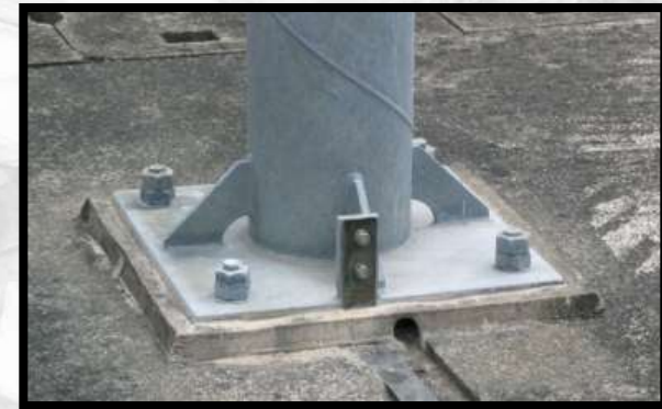
Void is filled with Sikadur 32 Hi-Mod
