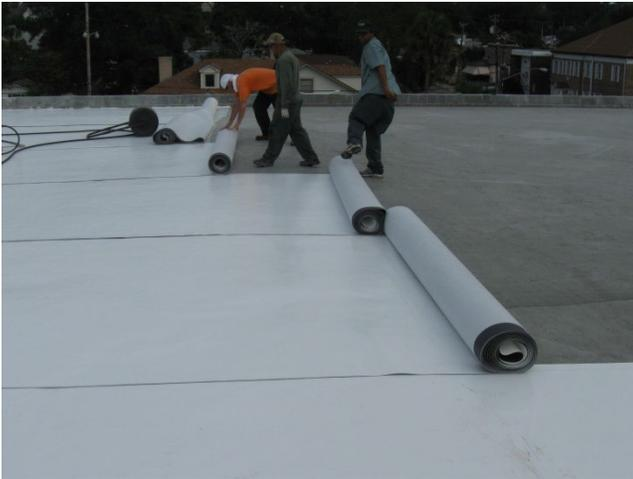
By rolling the membrane back evenly there is very little chance of dry laying the sheet as brooming and weighted rolling can follow immediately behind the sheet while the adhesive is wet. This method requires fewer workers to install and is also less likely to induce air bubbles compared with pulling the sheets back onto the other half.
