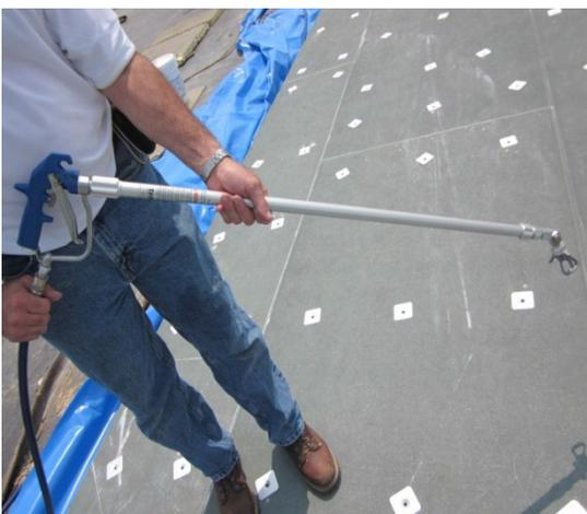
An extension wand can be added to most guns to make spraying more comfortable and to keep the spray away from the operator. A swivel tip allows for proper angling of the spray pattern.
