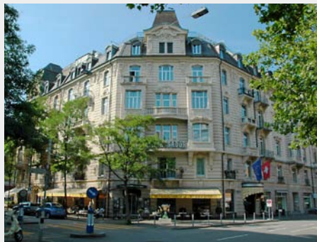
Hotel Ambassador Switzerland: Waterproofing and refurbishment solutions
