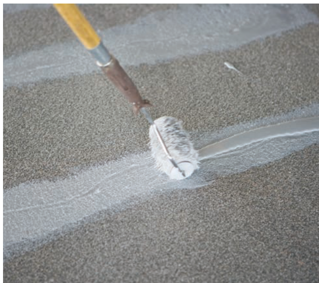
Detailing cracks
