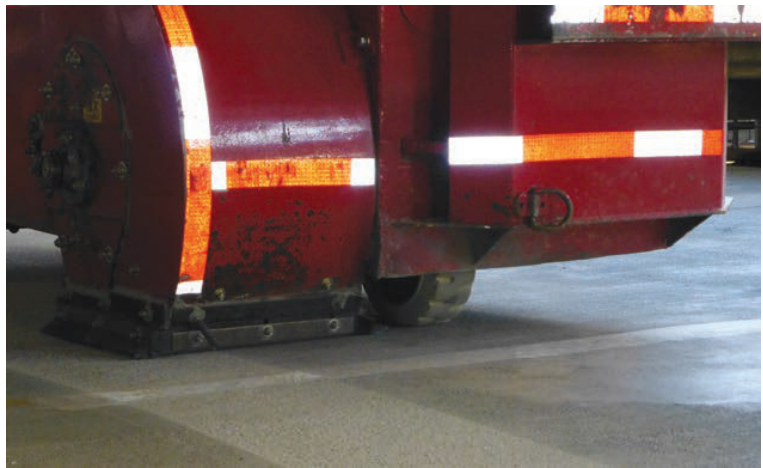
Shotblasting a concrete substrate
