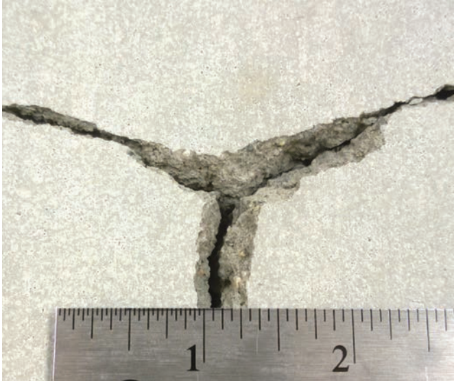
A. Improper detailing
