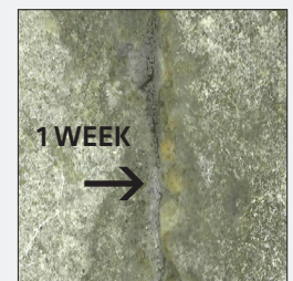
SikaControl®-245 WT Liquid Sealed Hairline Crack
