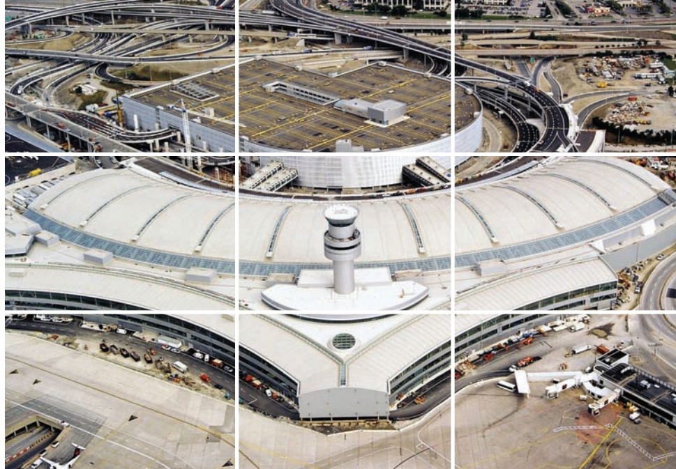
The Lester B. Pearson International Airport Terminal 1 in Toronto was designed through a joint venture consisting of three architectural firms — the facility was roofed by three roofing companies over a four-year period.
