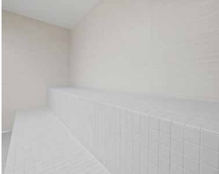
Snow White SikaTile®-825 Epoxy Grout and SikaTile®-815 Secure Grout blend with the steam room's tile. service level of its solution provider and the quality of the materials underneath," Carroll stressed. "Bryan and his team unquestionably supplied that first component, and we are proud to prescribe a system solution that addressed the Bocaire Country Club's unique conditions."
