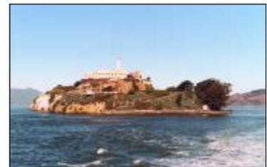
What most people do not realize is that the Alcatraz Cellhouse, the most visited and prominent building on Alcatraz Island, was also the largest reinforced concrete building in the world at the time of its completion in 1912. It was reinforced with "Ransome" bars, a patented square and twisted style of rebar that was sometimes used in the early 20th century concrete buildings.
