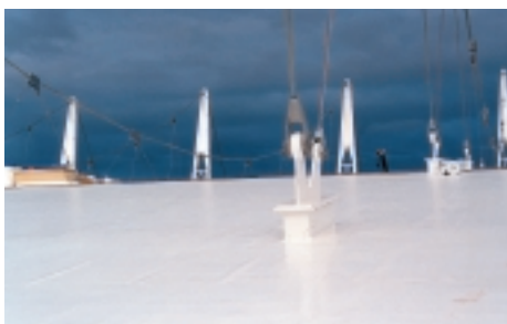
Steel cable attachment to Olympic Oval roof.
