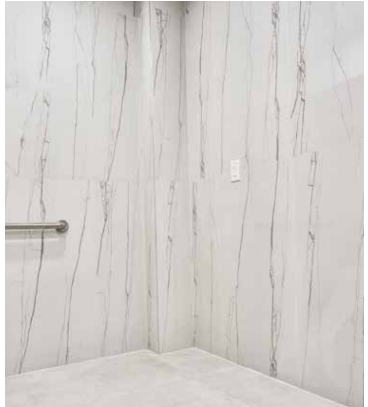
SikaTile®-400 LHT Pro Set was chosen for the first-floor bathroom due to its flexibility.
