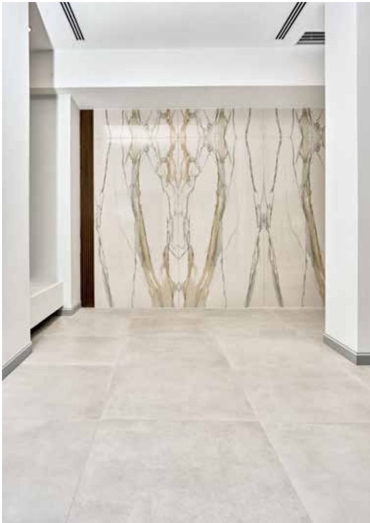
PIF set a variety of gauged porcelain tiles, panels and slabs for the $1.2 million redesign.
