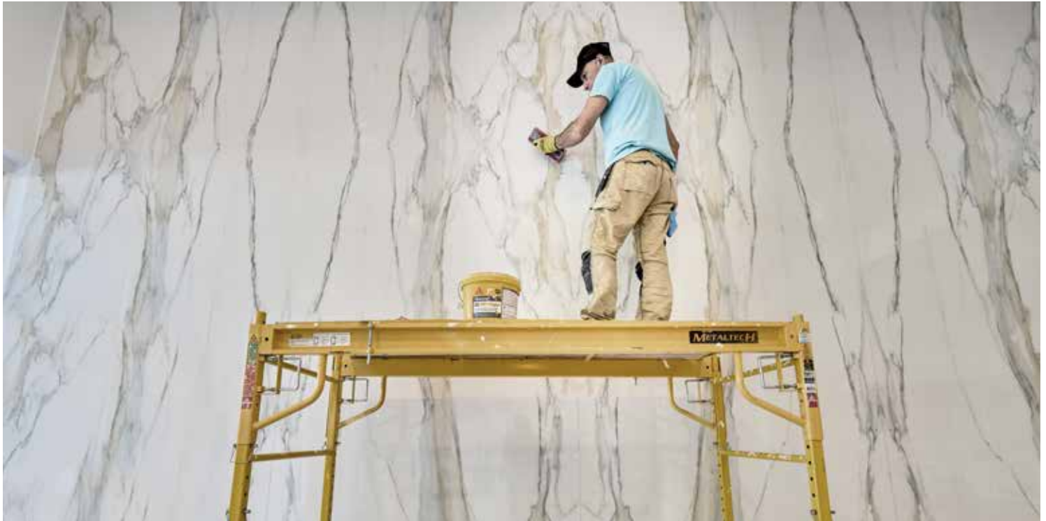
PIF's Grigorios Tsiknidis applies SikaTile®800 Unsanded Grout to huge Calacattaslabs.
