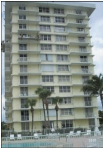
Concrete spalling primarily at the balcony edges and to a lesser extent at the walkways led to an investigation involving visual assessment and sounding to define areas of delamination. The analysis indicated that the quality of the concrete cover was poor and in many areas insufficient in depth. The building is also situated in an aggressive environment. The climate is hot and humid.
