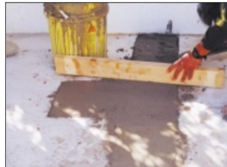
1. Remove delaminated concrete and apply Sika Armatec 110 EpoCem to all exposed reinforcing steel. Sika Armatec 110 EpoCem is a combination bonding agent and anti-corrosion coating. Because of its effectiveness to protect reinforcing steel, Sika Armatec 110 EpoCem is often used in locations where there is insufficient cover as a means of providing additional effective concrete cover.
