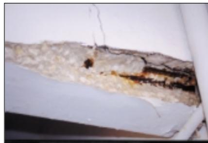
The buildings close proximity to the Atlantic Ocean makes it susceptible to intrusion of chloride ions. All of these factors contributed to accelerating corrosion of the reinforcing steel which led to spalling of the concrete at various locations along the balcony edges and walkways.
