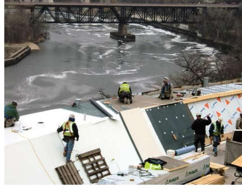
Obviously safety was also a concern. "We had to have the crew totally tied off to work on half of the roof, with no parapet walls and no curtain wall in that area," Hegge stated. "We also had to secure the crew against wind gusts created when the wind came down the Mississippi River."
