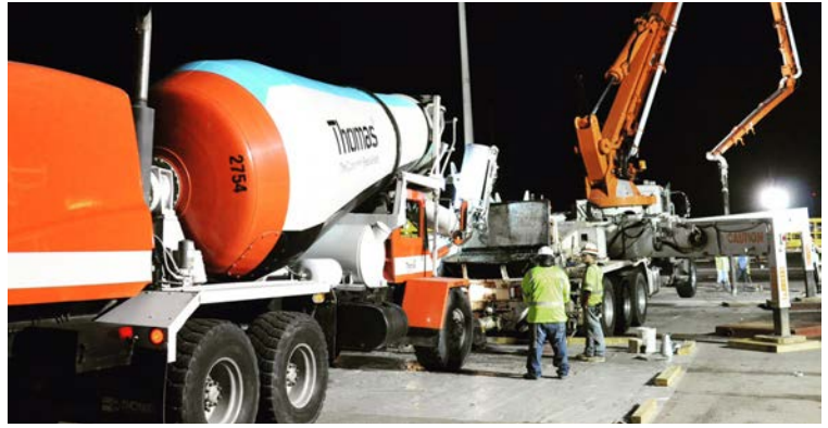
Thomas Concrete provided the concrete during the repair process
