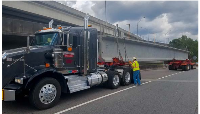
Prestressed concrete girders were brought in for the repair
