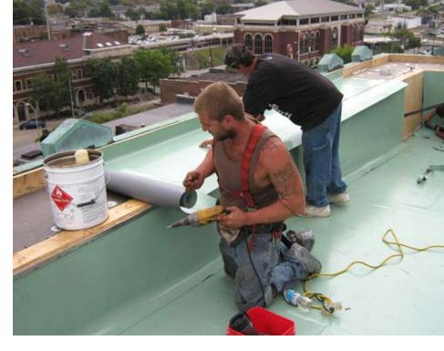
using Sarnacol 2163 adhesive. The patina green Sika Sarnafil membrane was then installed. "There was very extensive hand welding involved with the copper cornice flashing, and all flashings were field fabricated because of the color membrane," Randles pointed out.
