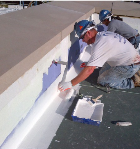
Step 4 - Detailing/Flashing
