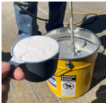
1 cup booster per 3 gallon pail of sealant
