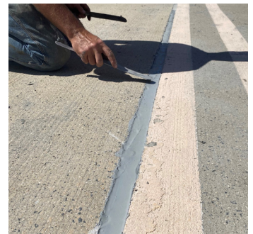
Tool/ Finish joint- 4 hours to cure!
