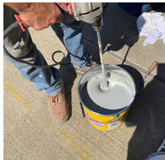
Mix 3 minutes with standard 2c mixing paddle
