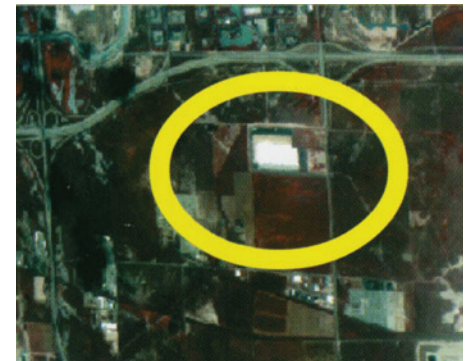
Figure 1: The R.C. Wiley Furniture Warehouse, Salt Lake City, clearly is visible in this aerial photograph.
