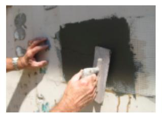
**4.** For base coats it is recommended to allow 48 hours cure time; for Senershield products 24 hours of dry time is recommended prior to pull testing. See photo.
