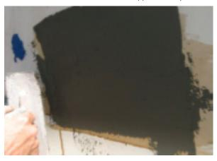
3. For the base coat, embed a 4" wide strip of Flexguard 4 reinforcing mesh into wet material; for Senershield products embed 4" SikaWall Sheathing Fabric into the wet material. Additional base coat or a Senershield air barrier can be applied to ensure full embedment. Use sufficient mesh or Sheathing Fabric so that 6" is embedded and 6" is left exposed for a pull tab.
