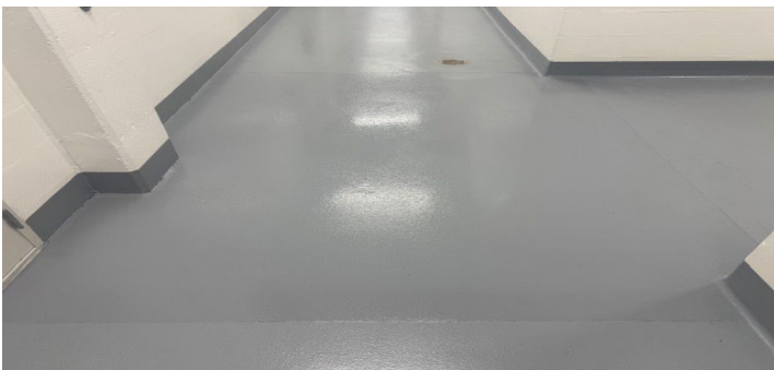
Corner detail showing integral cove base continuity.
