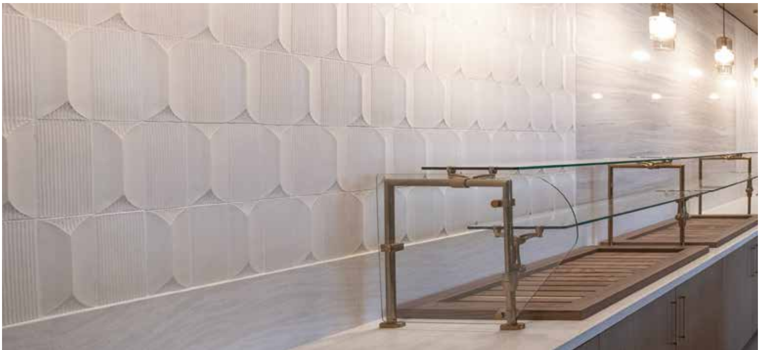
SikaTile®-400 LHT Pro Set secure more than 12,000 sq. ft. of tile at Ritz-Carlton, Naples.
