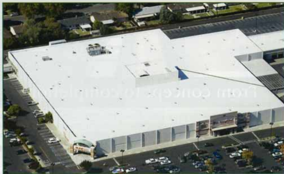
Photo 1 – 120,000-sq.-ft. retail project in which the original PVC roof was recycled into new membrane.
