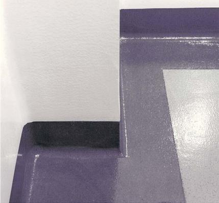
The technologically advanced Sikagard wall system from Sika offers smooth, seamless environments. By wrapping or tying the wall and ceiling into the floor and base and by rounding inside corners, the cracks and crevices that commonly harbor dirt and encourage bacterial growth are eliminated. The result is a seamless, aesthetic, hygienic surface that is easy to clean and maintain.
