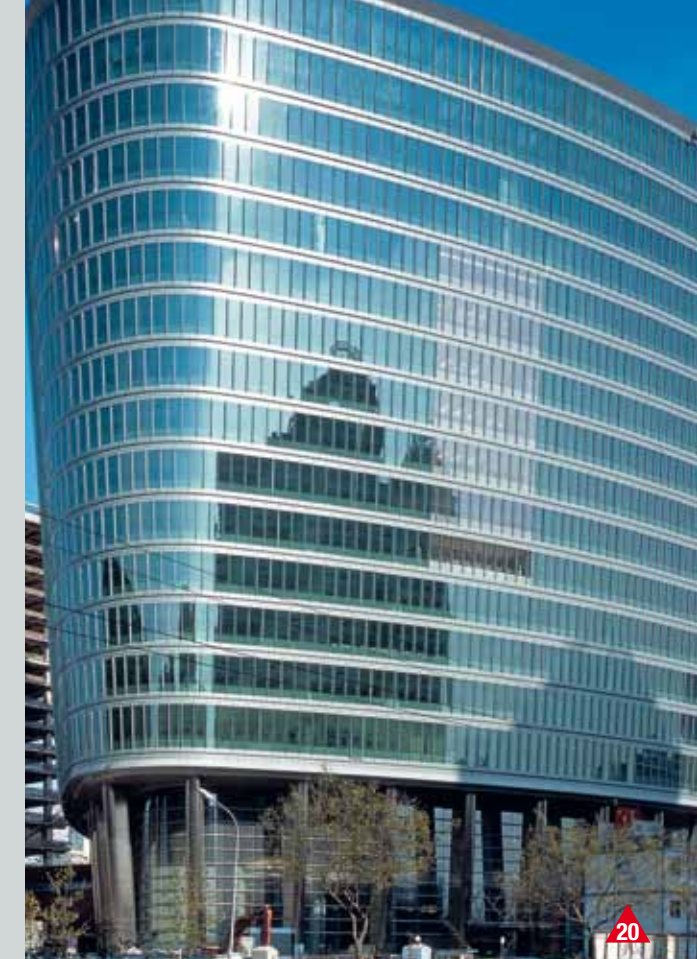
CNOOC Building, Beijing, China; Kohn Pedersen Fox Associates PC
