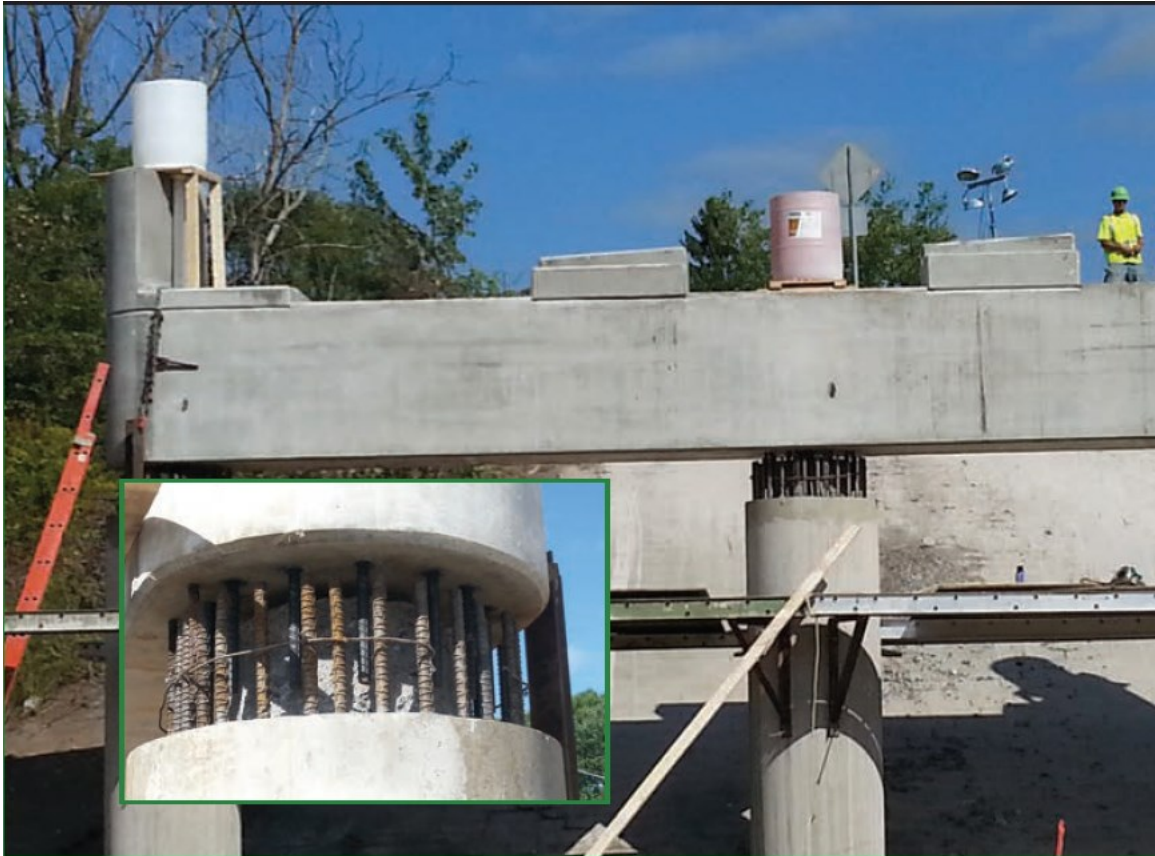
Lap-spliced substructure. Hooper Rd. Bridge Union, NY Ref: FHWA
