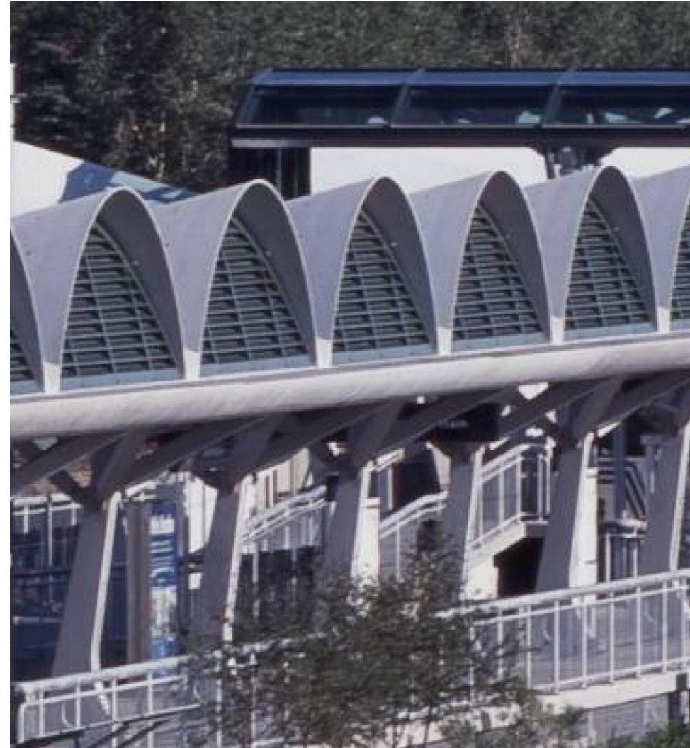
Shawnessy Light Rail Station Canopy Roof Calgary AB
