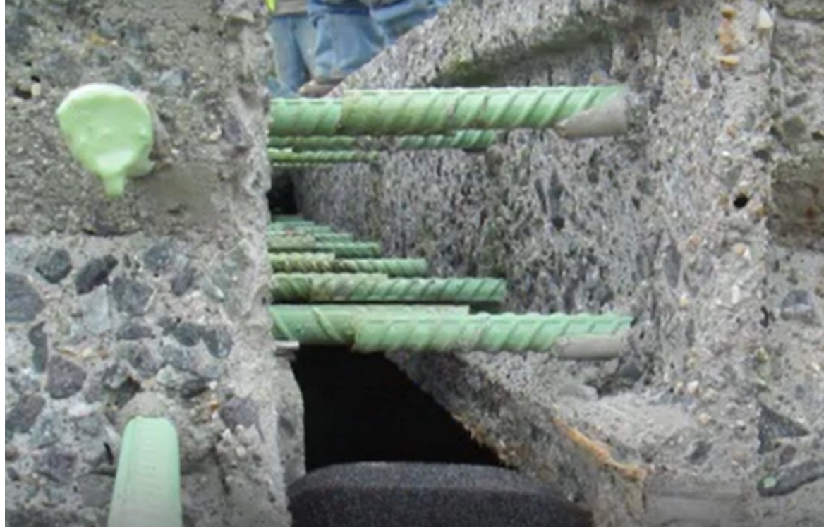
Pre-fabricated bridge deck panel connections
