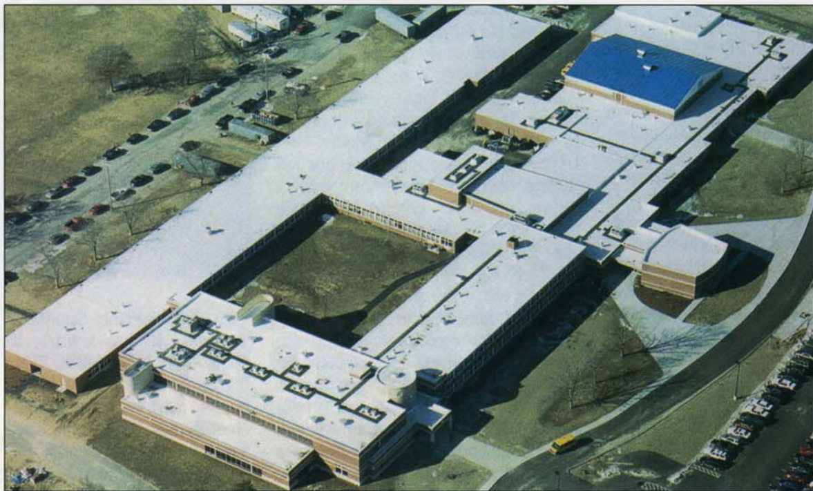
Capeway Roofing Systems, Westport, Mass., reroofed the Apponequet Regional High School in Lakeville, Mass. On the low-slope deck areas, Sarnafil's white G410 EnergySmart membrane was adhered to insulation panels with a low-odor, low-VOC, water-based adhesive. On the steep-sloped portion over the gymnasium roof, Capeway installed the Décor profile over the G410 membrane, both in azure blue.
