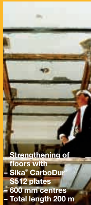
Installing the Sika® CarboDur® S512 plates
