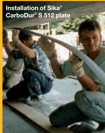
Soffit of strengthened bridge
