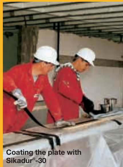
Easy installation of Sika CarboDur plate
