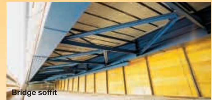
Application of Sika® CarboDur® plates
