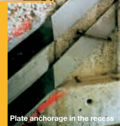
Configuration of CRP plates on the load-bearing masonry wall
