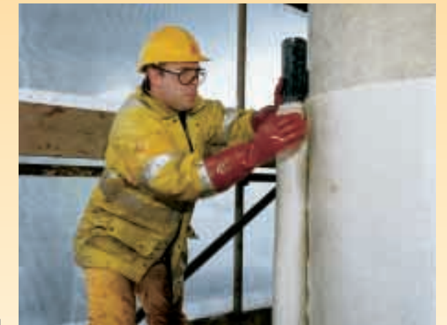
Application of SikaWrap® Fabric System for impact resistance on a bridge column
