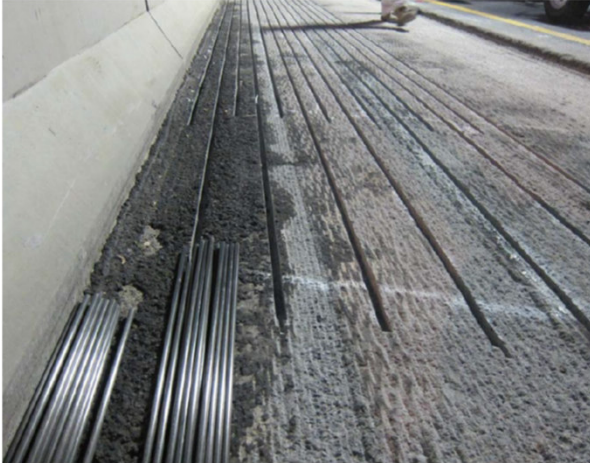
Cut and clean grooves
