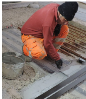
Apply adhesive (if bonded)
