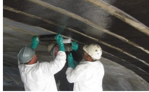
EXTERNALLY BONDED FRP OR STEEL
