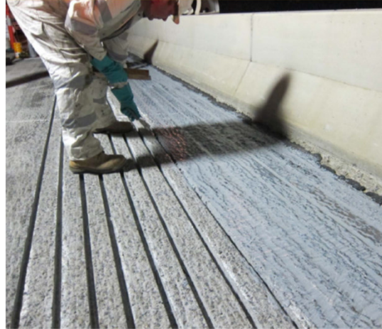
Place rods in the groove
