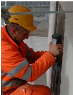
Installation of tendon
