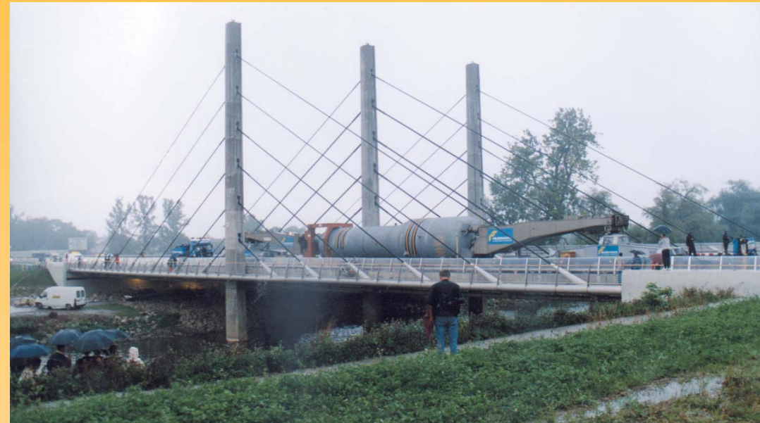
Heavy Truck Crossing the Bridge
