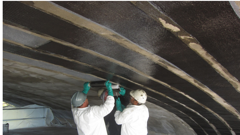
SikaWrap® systems are effectively used in strengthening of bridges.
