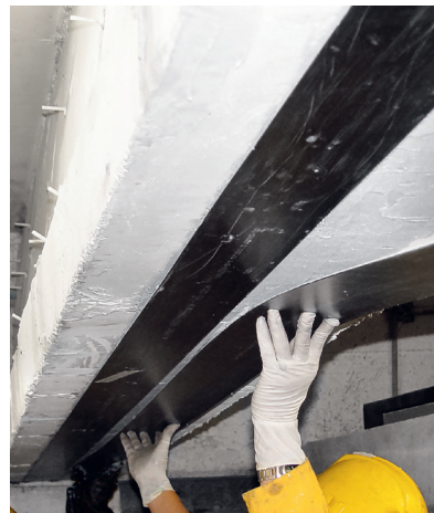
CarboDur® laminates are commonly used to reinforce concrete beams.
