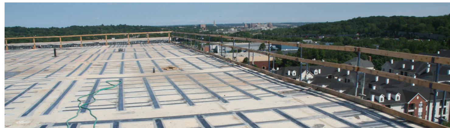
CarboDur® laminates are applied for top strengthening of slabs which can be coated and finished to desired finish.
