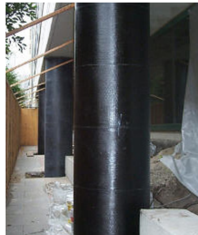
SikaWraps' conformability are ideal for column strengthening.
