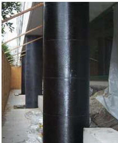
SikaWraps' conformability are ideal for column strengthening.
