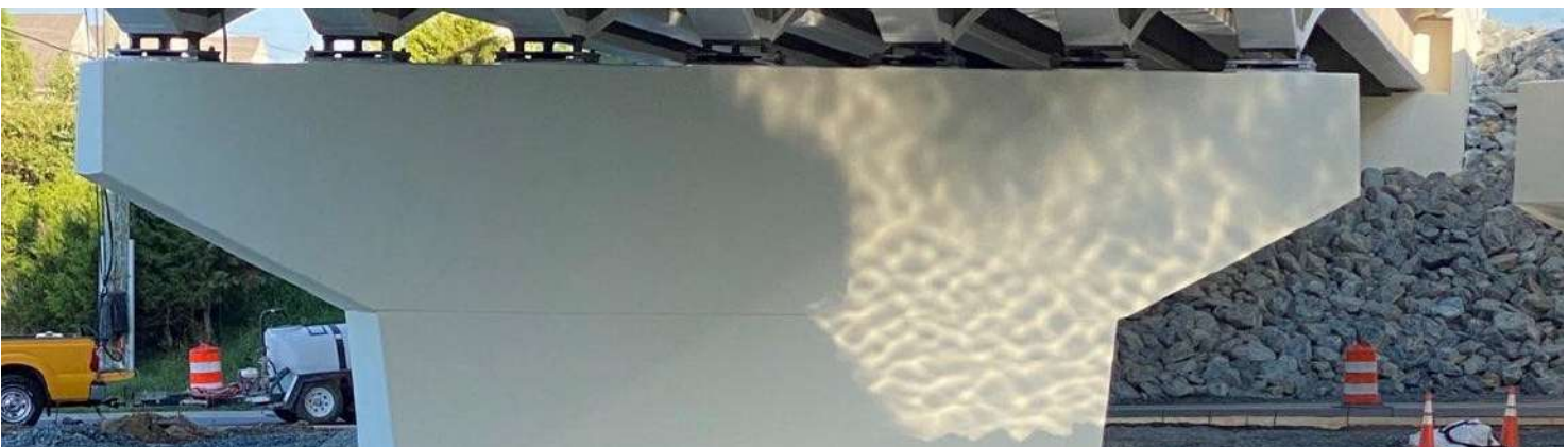
Sikagard® products can be applied as a top-coat to SikaWrap and CarboDur systems in hundreds of standard colors to protect them from UV and weathering exposure.
