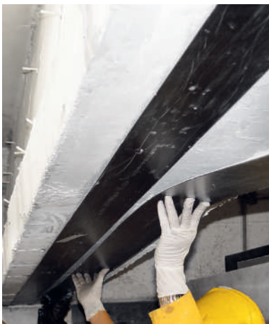
CarboDur® laminates are commonly used to reinforce concrete beams.
