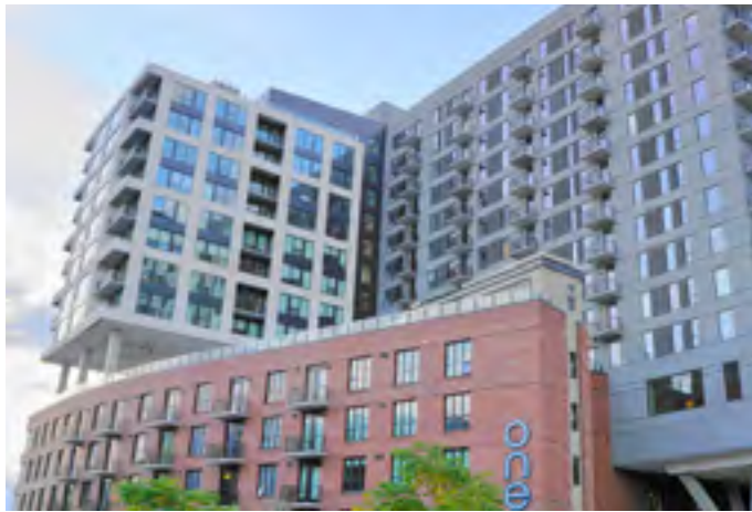
Panelized EIFS One Seven at Belleview Station Denver, Colorado
