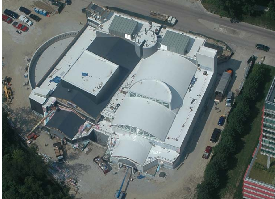
A view of the Holocaust Museum while under construction. A Décor Roof System was installed by A-1 Roofing of Elk Grove IL. The facility's unique design called for a roof consisting of varying angles, two distinct colors and both a barrel and gable roof.
