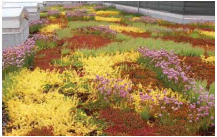
Tri-City Wastewater - Oregon City, OR
