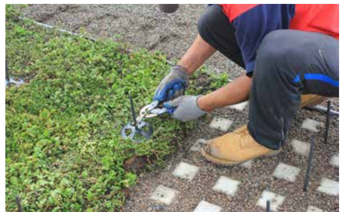
Vegetation installation is completed with trimming of Disk Anchors
