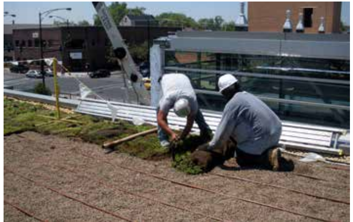
Plant materials being installed over prepared LiteTop®
