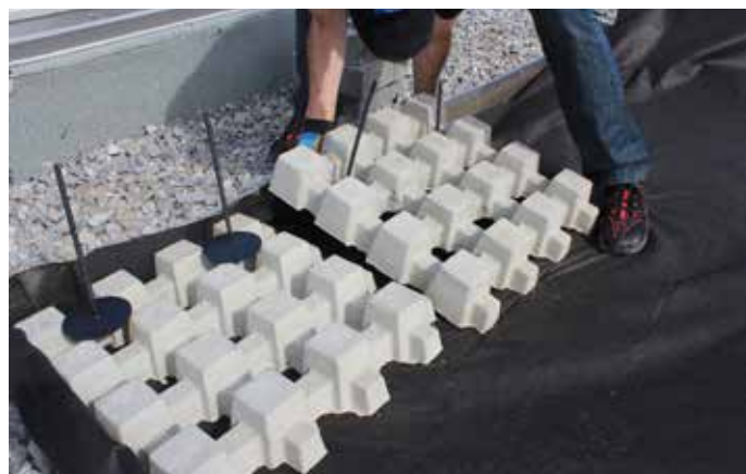
Checker Block® installation on rooftop
