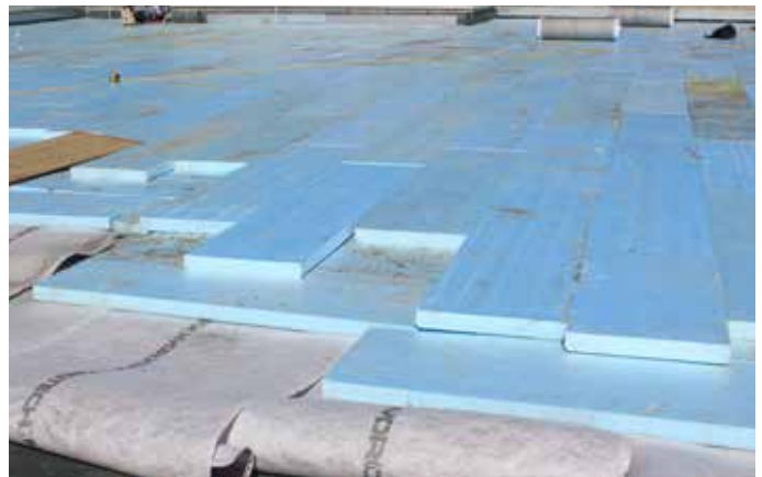
DuPont STYROFOAM® is installed in layers to depth needed to achieve R-rating
