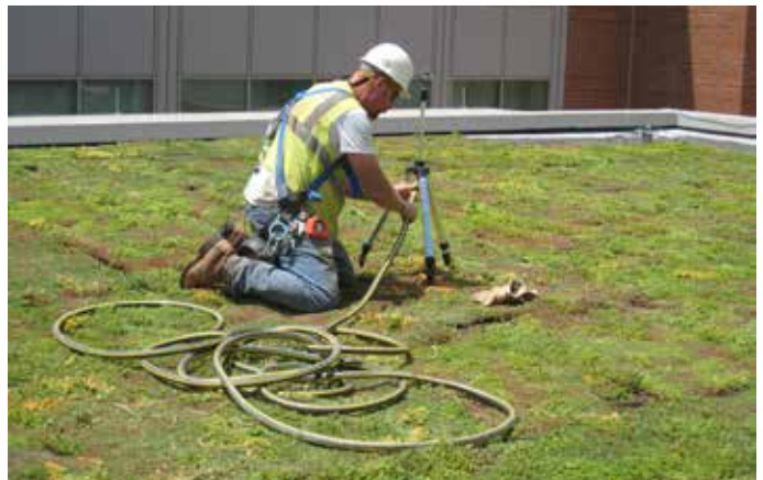
Irrigation being readied for new Garden Roof® planting
