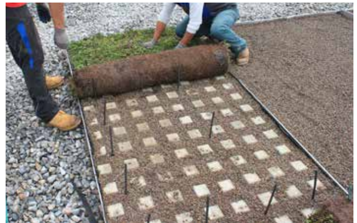
InstaGreen Carpet installation over Checker Block and Disk Anchors
