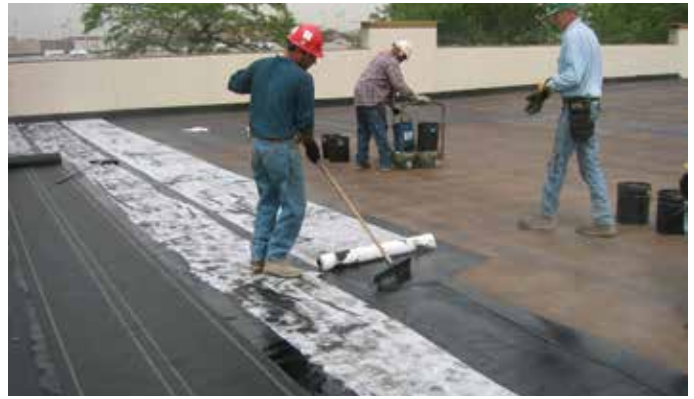
Installing MM6125-FR waterproofing membrane with reinforcing fabric - total thickness of 215 mils
