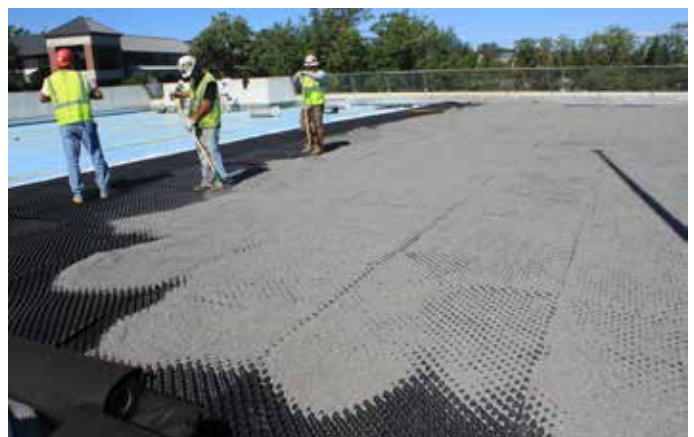
Gardendrain® installed over insulation and filled with lightweight aggregates (optional)
