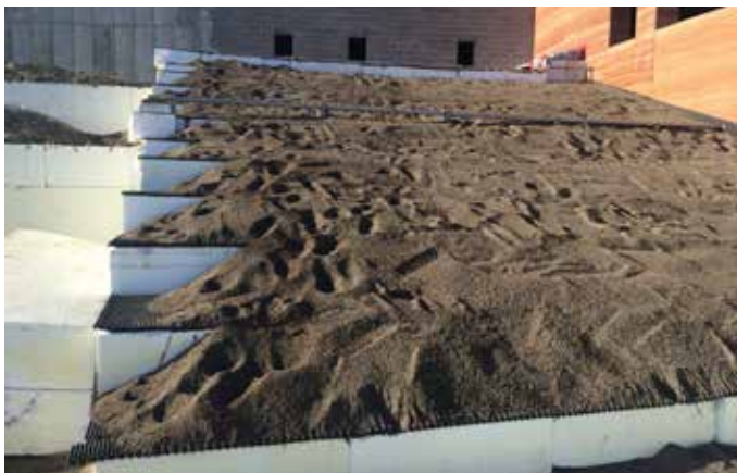
Stepped geofoam used to create topography - Brinton Museum - Brinton, WV
