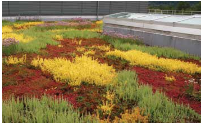
Tri-City Wastewater - Oregon City, OR
