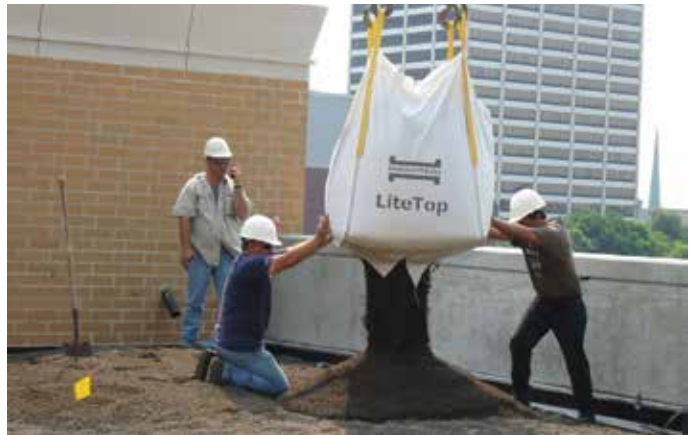
LiteTop® installed to desired depth
