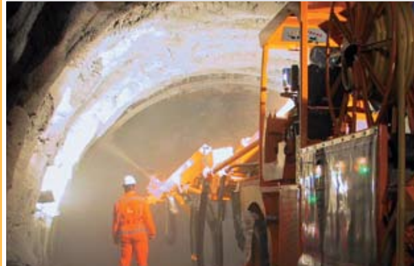
Sika-PM500 shotcreting system for large sections
