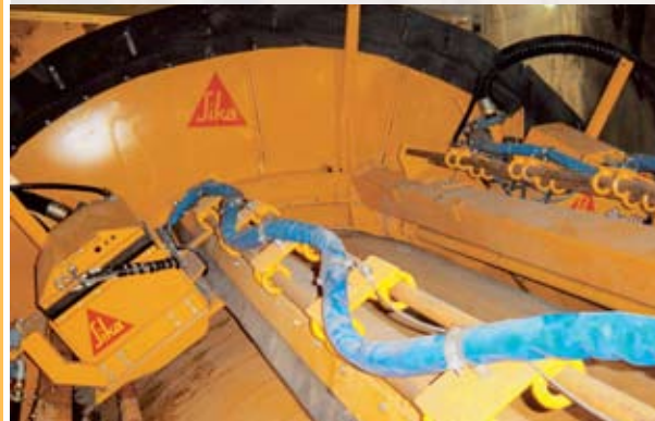
Shotcrete stabilization in TBM heading
