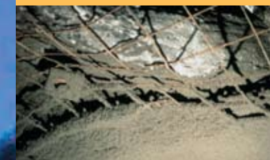
Concrete spraying, spraying shadow/rebound 2
