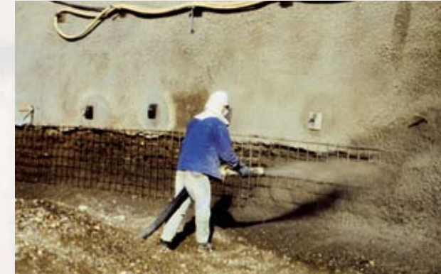
Excavation stabilization
