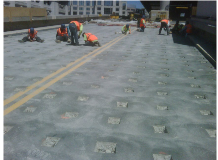
Union Station Ramp, DC 2010
