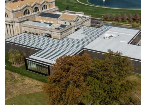
All of this work was done during winter, which required storing roofing materials in the recently completed underground parking area and using heaters to keep the materials warm and ready to be used as needed.
